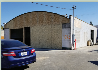
Construction begins for Sac Yard Tap House & Biergarten at 1725 33rd Street.
